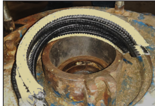
DualPac 2211 cut rings were installed.
